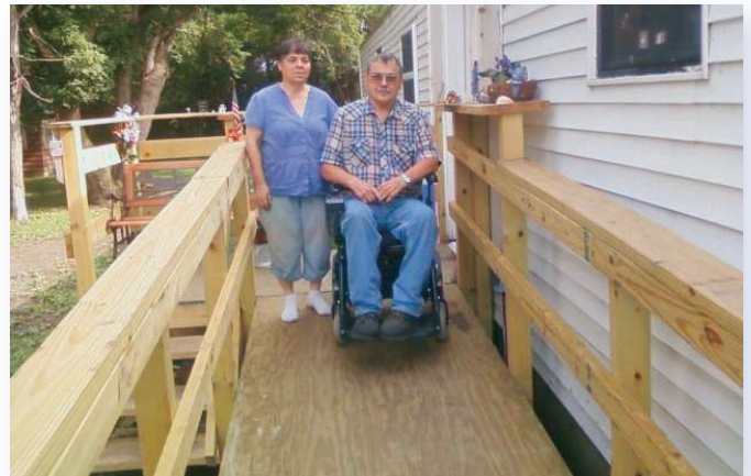
Ronnie Wagner with the new wheelchair ramp into his home.
